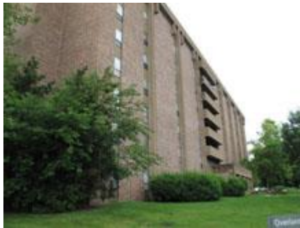
Overland Towers Apartments Overland Park, KS
