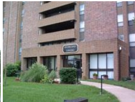
Overland Towers Apartments Overland Park, KS
